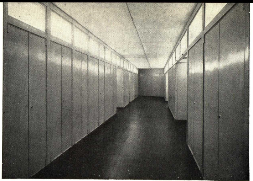
Fig. 19. A view of one of the main corridors of the C.P.D.E. building, showing Snead Type "SFS" all steel to 7 ft. with glass above to ceiling
