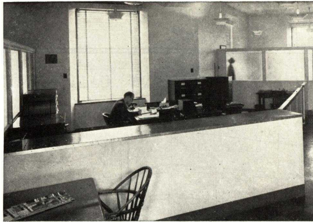
Integrally built-in counter with slide doors and shelves in rear. Linoleum top with white metal edging
