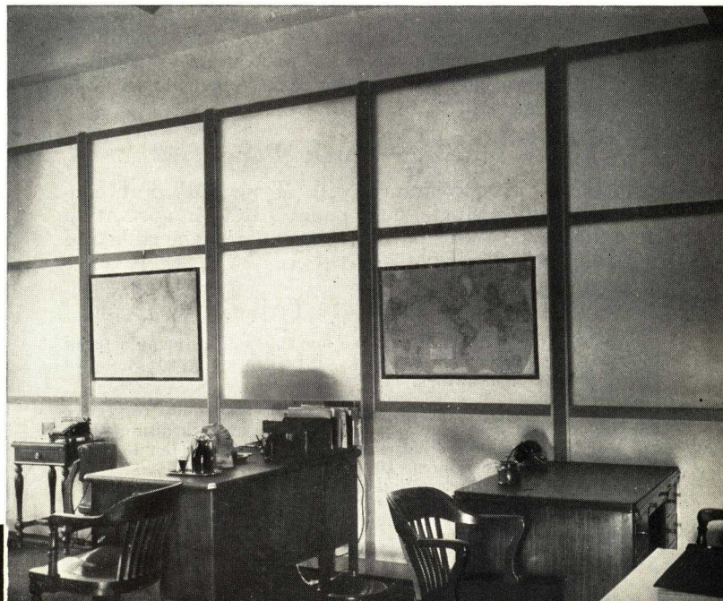
Right: Fig. 21. Both light and sound proofness are obtained here with a double-glazed wall of Type "SFS"
